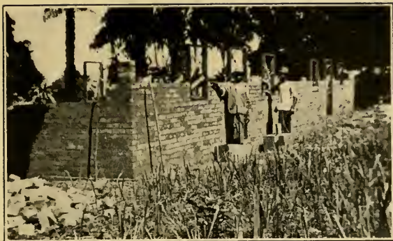
BUILDING BOYS' DORMITORY Tshumbiri
